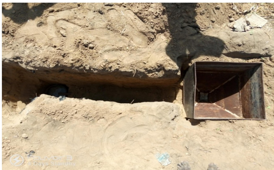
Plate 1: Installation of a Lysimeter
