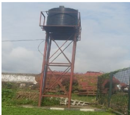
Plate 1: Vandalised Water Borehole at Ogale
