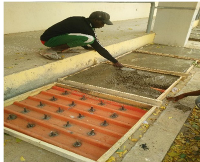
Figure 2. Casting being carried out in fully supported condition
