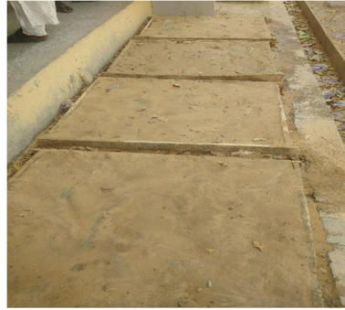
Figure 5. Curing of the slab
