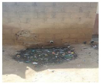
Plate 1: Cesspool for disposing grey water in water in Gamboru ward
